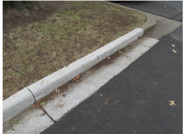
Recently replaced curb and gutter
