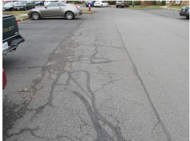
Bradwood Court pavement overview Note: Cracks and previously sealed cracks
