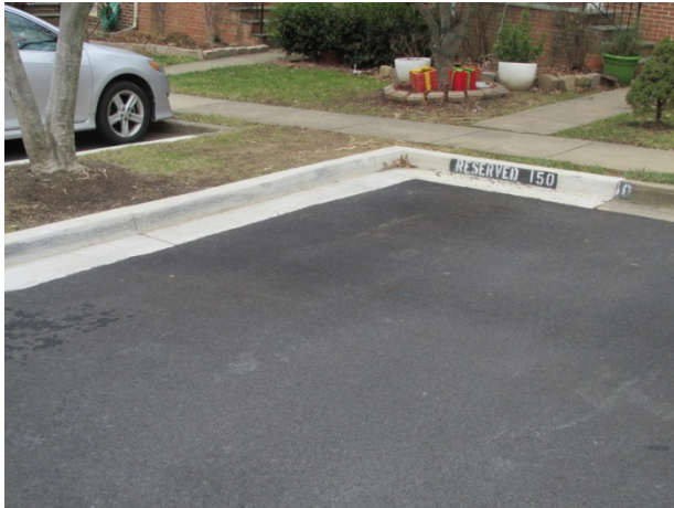
Recently replaced section of curb and gutter
