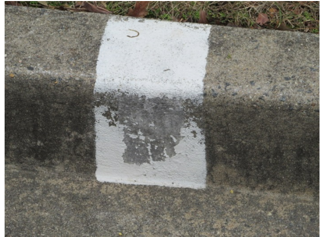
Curb paint finish deterioration
