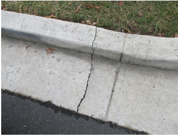
Crack at recently replaced section of curb and gutter
