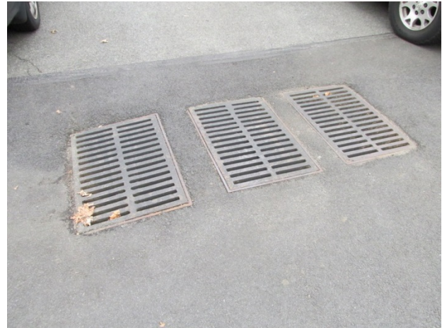
Minor settlement at catch basin inlets
