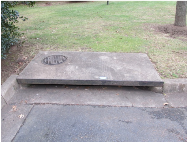
Typical curb inlet catch basin
